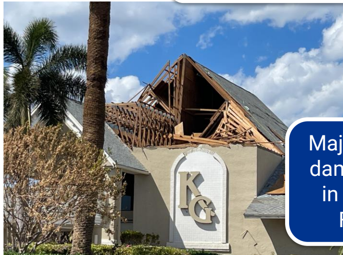
Wind damage to soffits, flashing in a high-end hotel in Cape Coral, FL
