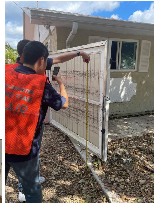
Between 5-7 feet surge high water marks in areas close to the bay
